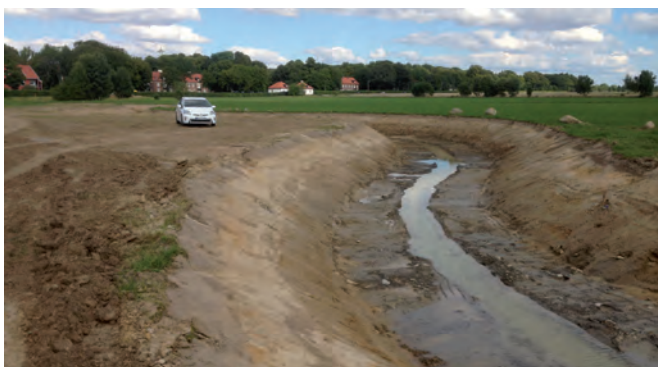
At Pålsjö a stream is excavated and recreated after many decades of being in a culvert.
