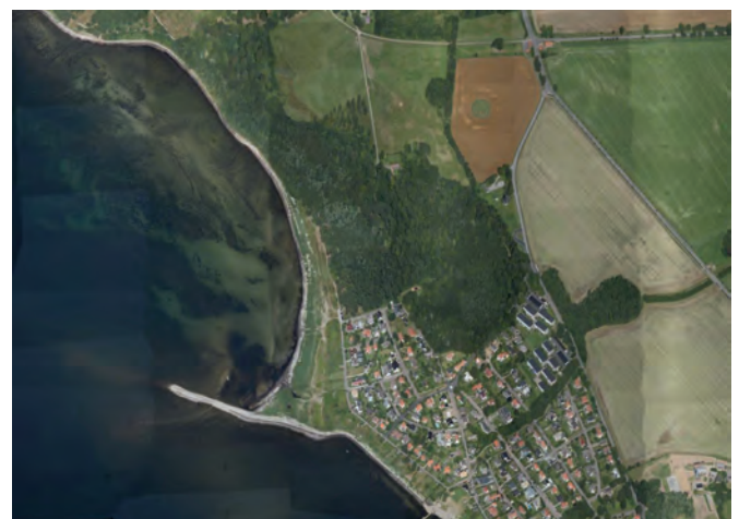
Part of the three main green corridors of the Helsingborg comprehensive plan. The small stone reef of Hittarp and the nature reserve Kulla Gunnarstorp forest are visible.
